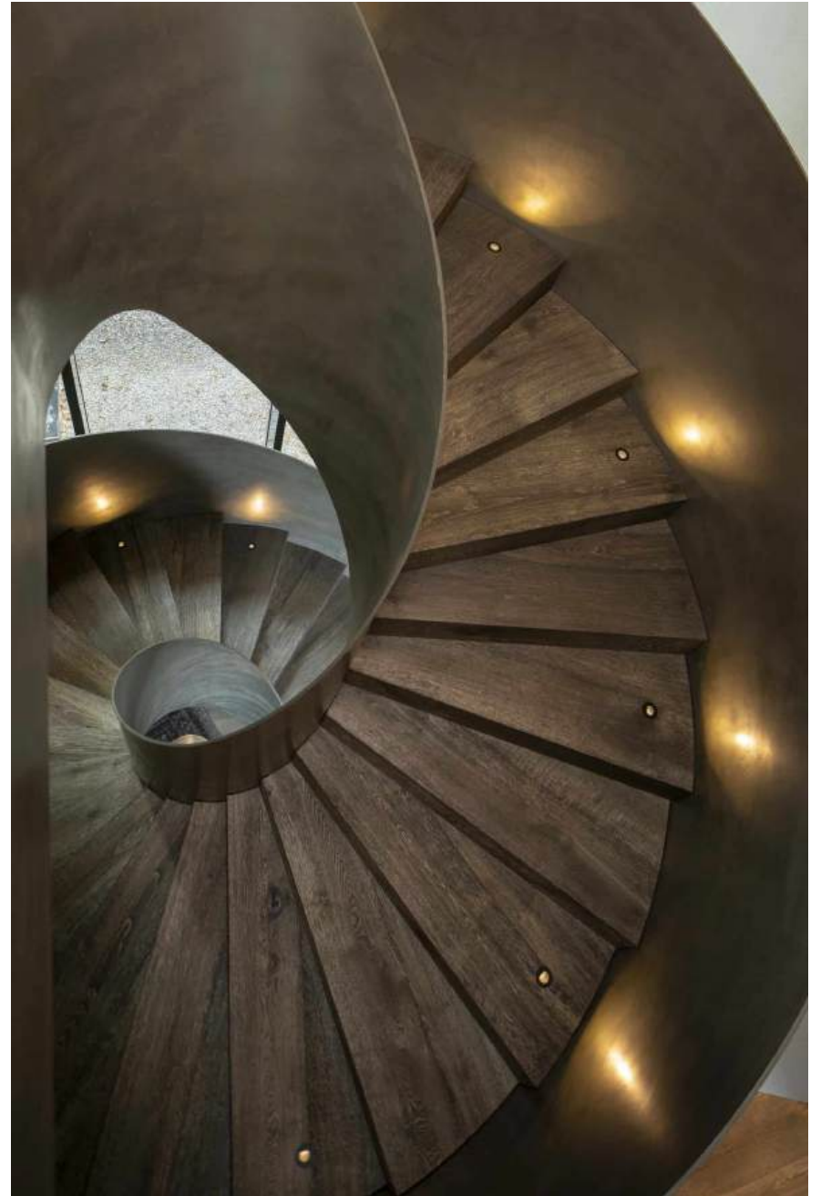
Project: Stairs in a private villa Design: AR Architektur Metal: VeroMetal Nickel-Silver Substrate: Steel
