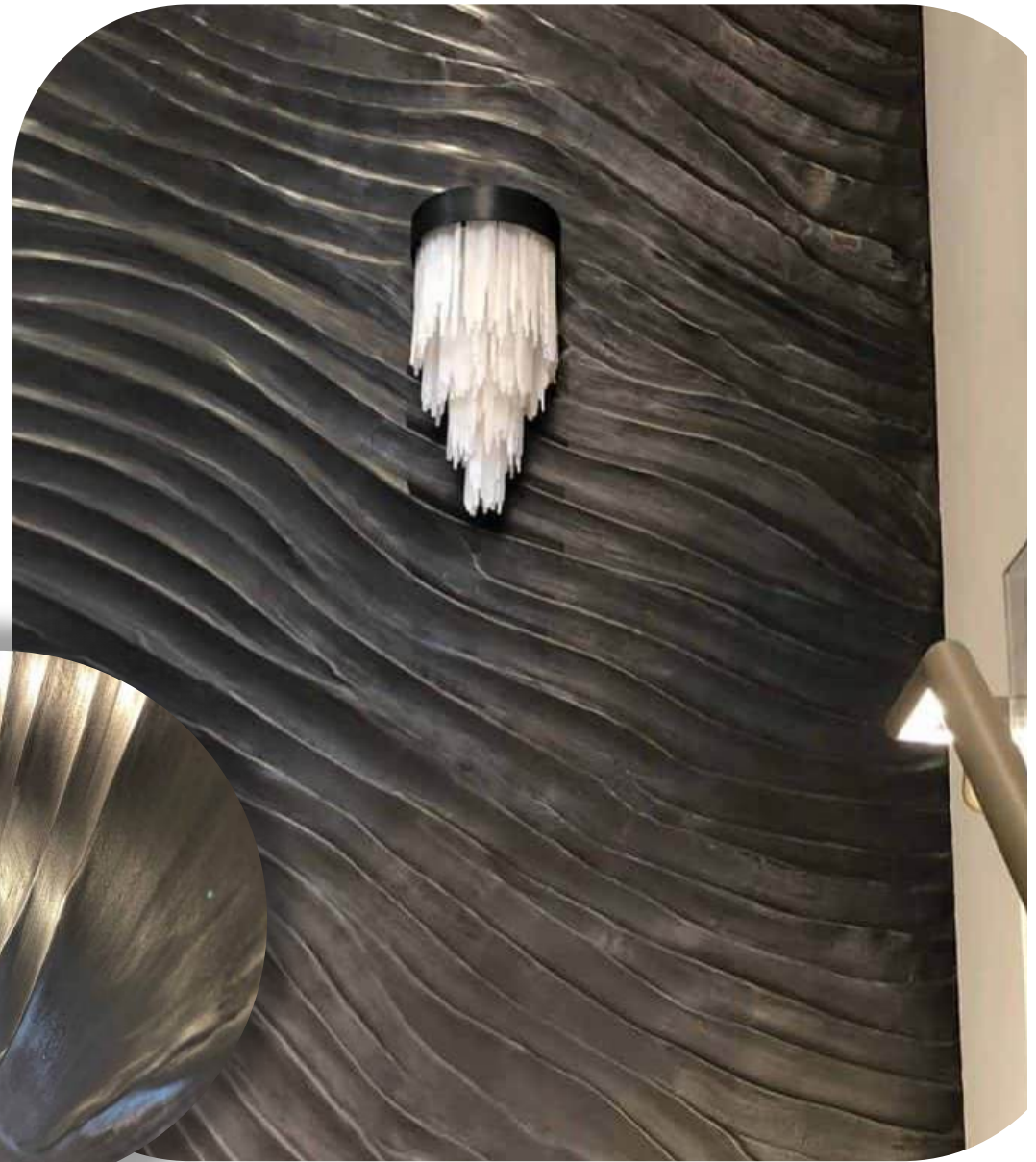
Project: Wave wall Metal: VeroMetal Manganese Surface: Black patina Substrate: Stucco
