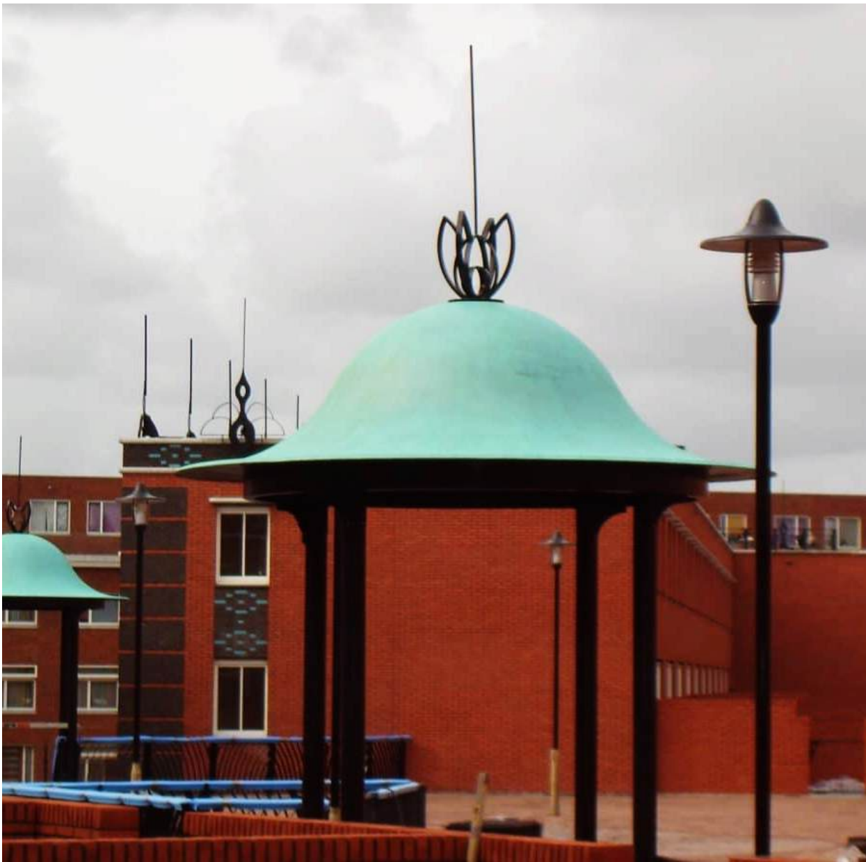
Project: Domed roof Design: Wam Architecten Metal: VeroMetal Copper Finish: Green patina Substrate: Polyester
