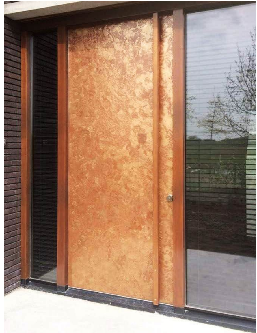
Project: Front door Architects: VDP Architecten Made by: ITS Polyester Metal: VeroMetal Copper Substrate: Multiplex
