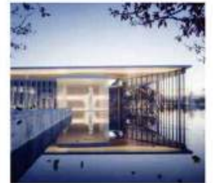
Each piece of art is the crystallization of towering thoughts. Under the light, its artistic beauty permeates the heart and soul, and instantly fills the space with inspiration. Rigart creates exclusive lighting aesthetics for the art space.
